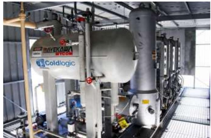
The basic concept of the AHP works on the basis that discharge gas from the high side of the ammonia refrigeration plant is drawn and recompressed by a high pressure compressor. This elevates the pressure and increases the temperature which in turn is passed through a heat exchanger where it transfers its heat to water on the other side.
