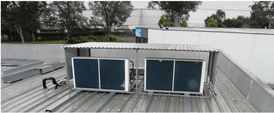
Figure 2 - Ideal installation of condensing units (source Minus40)
