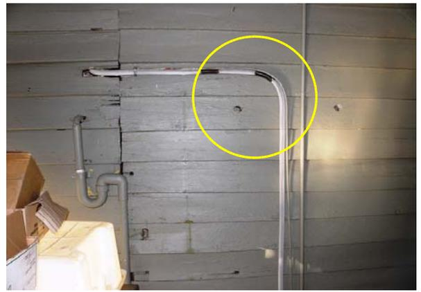
Figure 4 - No insulation, leading to ice formation (source – Minus40)
